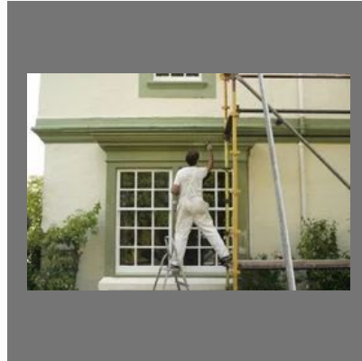
Exterior Wall Painting Service
